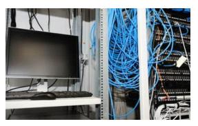
It is essential that space be provided for adequate computer/network wiring. All network wiring shall terminate in this room. It will also be the entrance point for the ISP. All electrical wiring will terminate in a separate designated room and the use of a raised floor is recommended.
